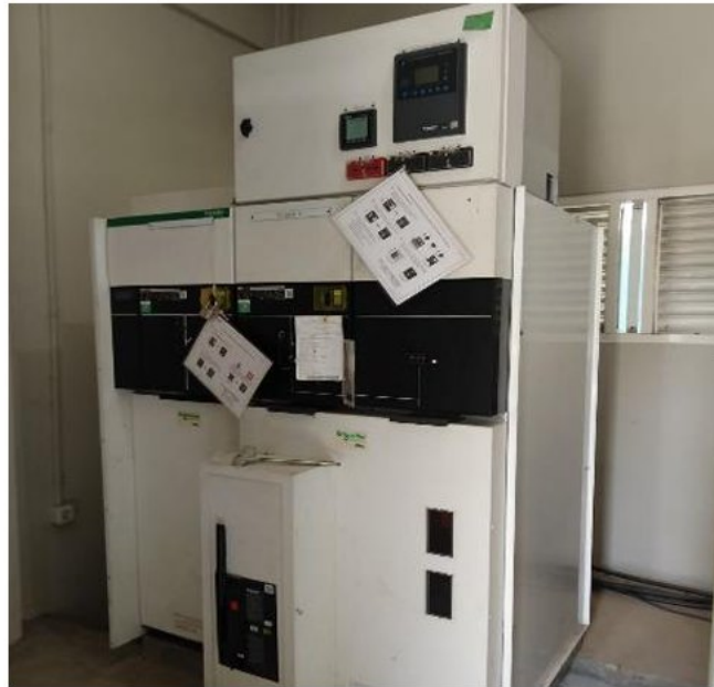
Figure 2 20kV Switchgear in the Campus Building
