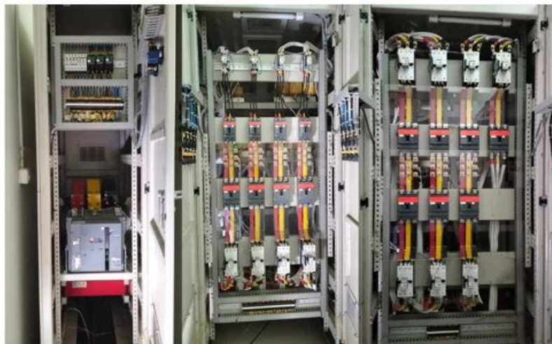
Figure 1 Capacitor Bank Panel
