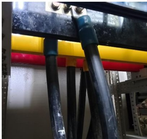
Figure 6 Result of cable installation on the main busbar of the LVMDP panel
