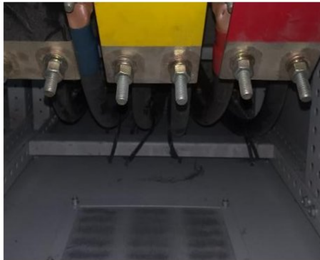
Figure 4 Incoming ACB cable before reduction
