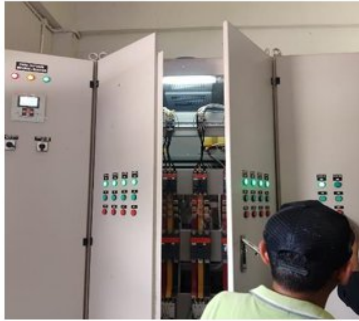
Figure 10 Testing the Control Installation Circuit
