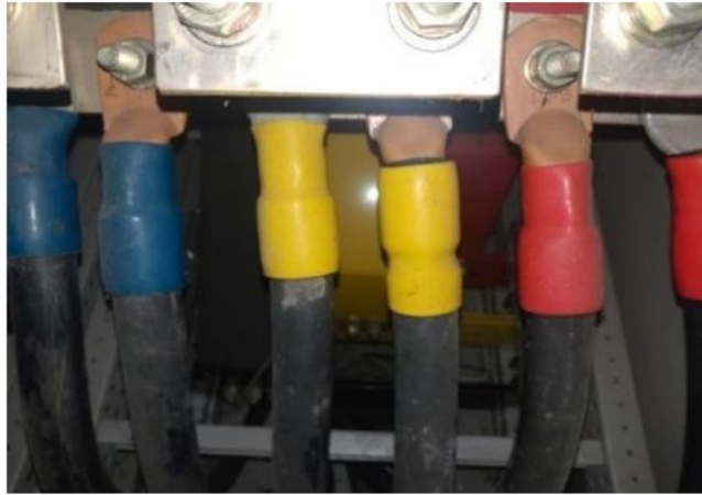
Figure 3 Incoming ACB cables before reduction
