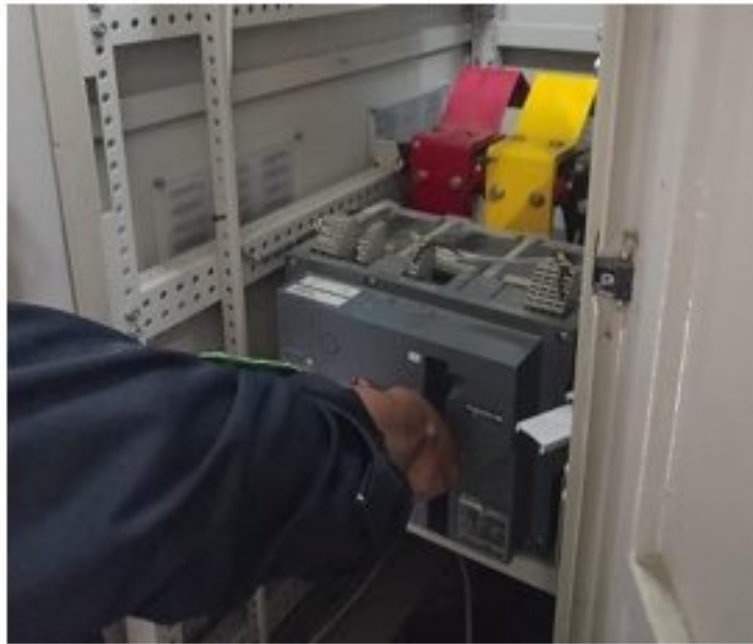
Figure 8 Activation of the Capacitor Bank ACB Panel
