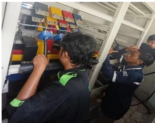
Figure 5 Cable installation process on the main busbar of the LVMDP panel
