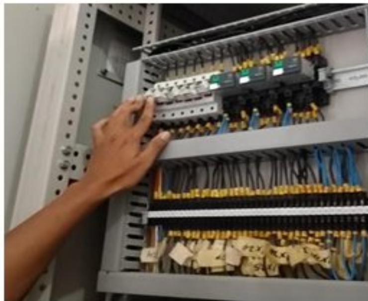
Figure 9 Activating the Fuse
